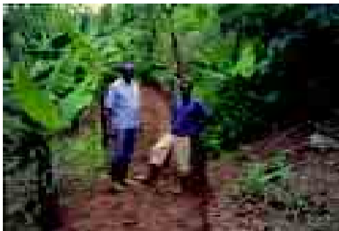
James standing in his newly constructed infiltration ditch: one of the most widely adopted techniques under the project
